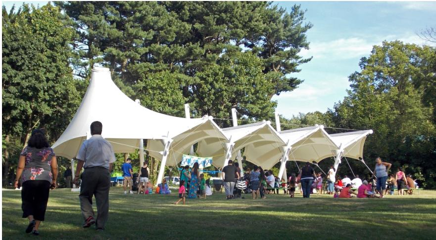
*The "Meadow Structure" pavilion features a tensile fabric roof with photovoltaic film attached to its upper side. Photo: Courtesy Marpillero Pollak Architects*
