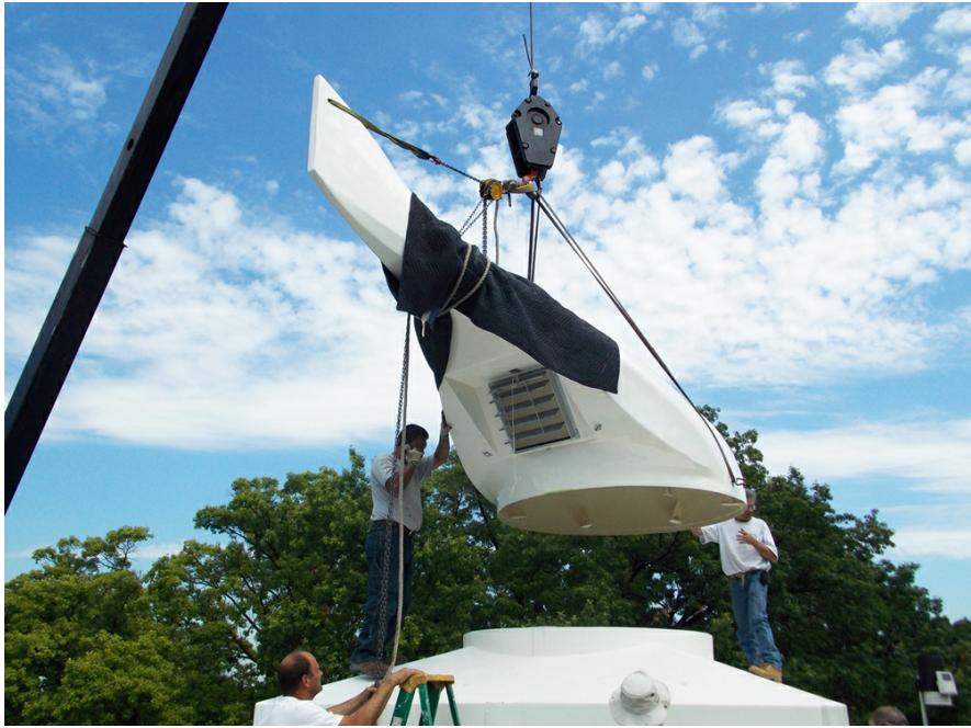
*A second skylight was retrofitted with a skylight windscoop that provides ventilation as well as daylight.*
